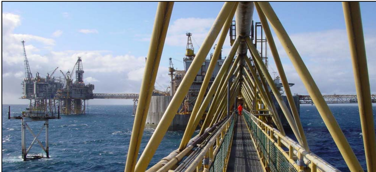
Flare bridge at Ekofisk.
